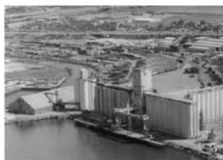
Bulk elevator, terminal and warehouse operations - Port of Stockton, California.
